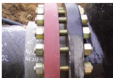
Figure 3. Flange joint [6]
