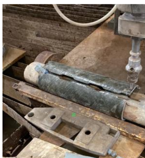
Figure 12. Pipe after cutting
